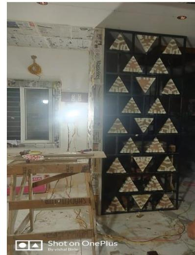
Now these triangle pieces are finished with 3 different types of laminates with the help of adhesive material.
